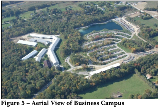
Figure 5 – Aerial View of Business Campus
