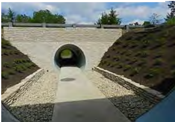
Muirfield Drive Pedestrian Tunnels
