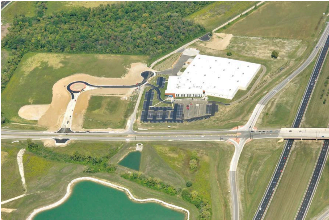
Motoman project with the connector road to the west of the Austin Interchange
