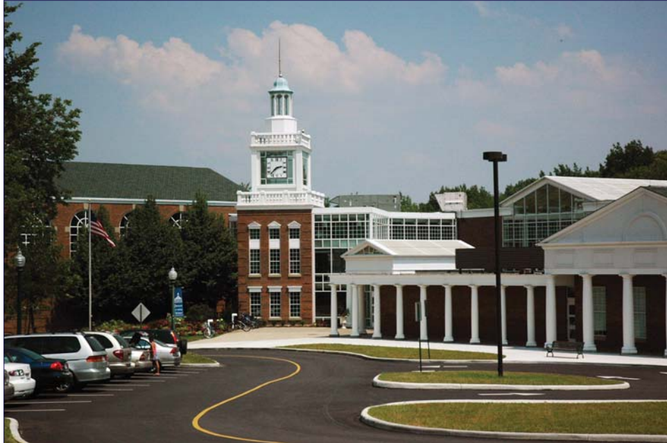
The completion of the Brecksville Community Center parking lot renovation.
