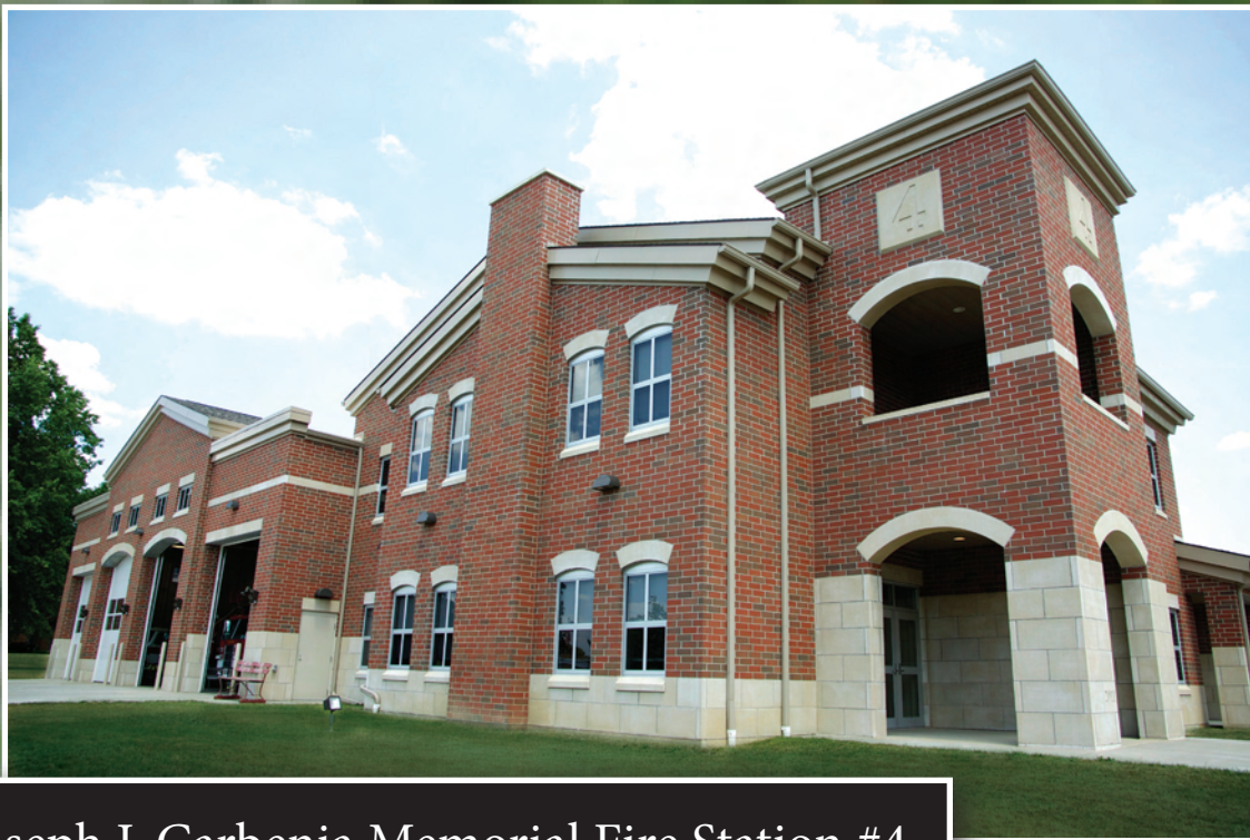
Joseph J. Carbenia Memorial Fire Station #4 City of Canton • 2504 Cleveland Avenue NW
