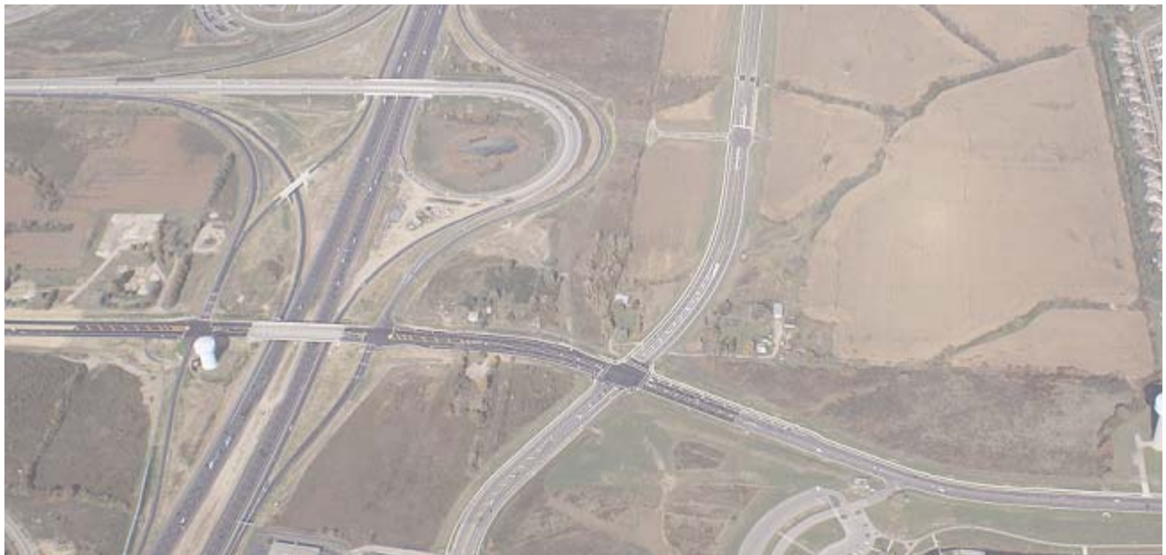
October aerial photograph of the Liberty Way interchange and development potential immediately adjacent to the interchange and the Cox Road extension.
