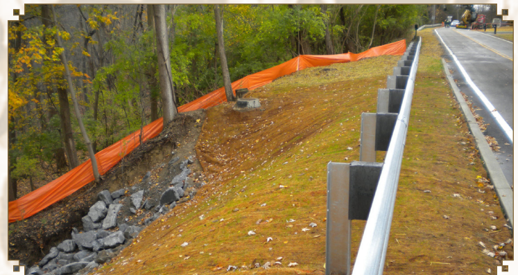
Greenhaven Road drainage improvements.
