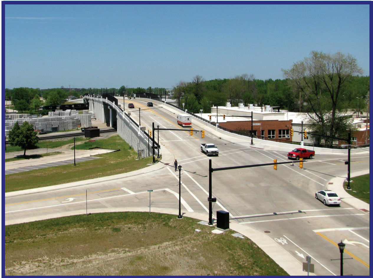
Front Street Overpass, North-end of Berea
