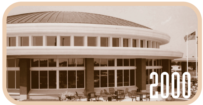
A view of the newly constructed Great Lakes Service Plaza. Reconstructing the original service plaza facilities is part of the Commission's Capital Improvement Program.
