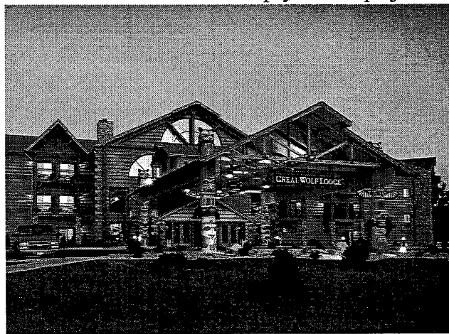
Construction on Mason's Great Wolf Lodge Resort, which includes an indoor water park, began in 2005.
