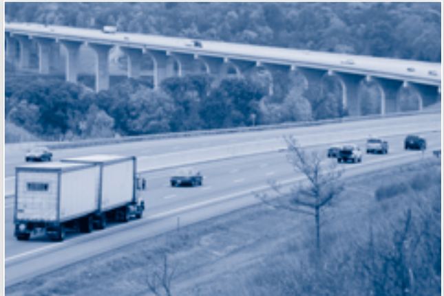
The new Cuyahoga River Bridges were opened in 2003 and provide a third lane for travelers.
