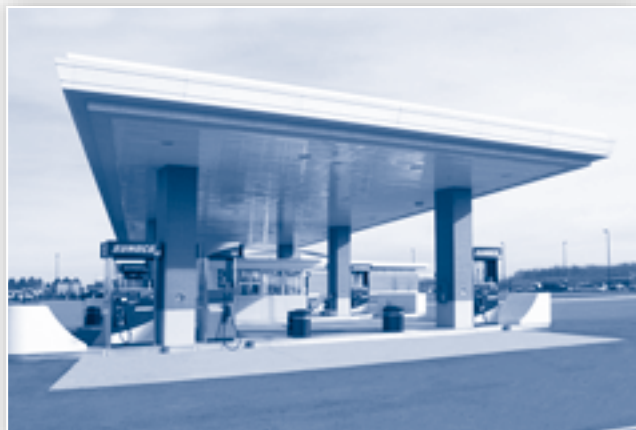
New fuel islands at the reconstructed plazas offer service to multiple customers.
