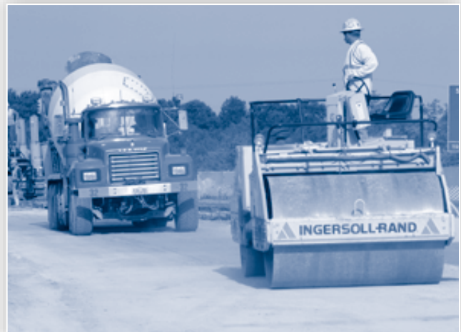
Ongoing construction for the State Route 58 Interchange (#140).
