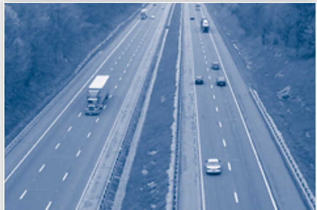
This portion of the Turnpike roadway shows a new third-lane section and a two-lane section which has yet to undergo construction.
