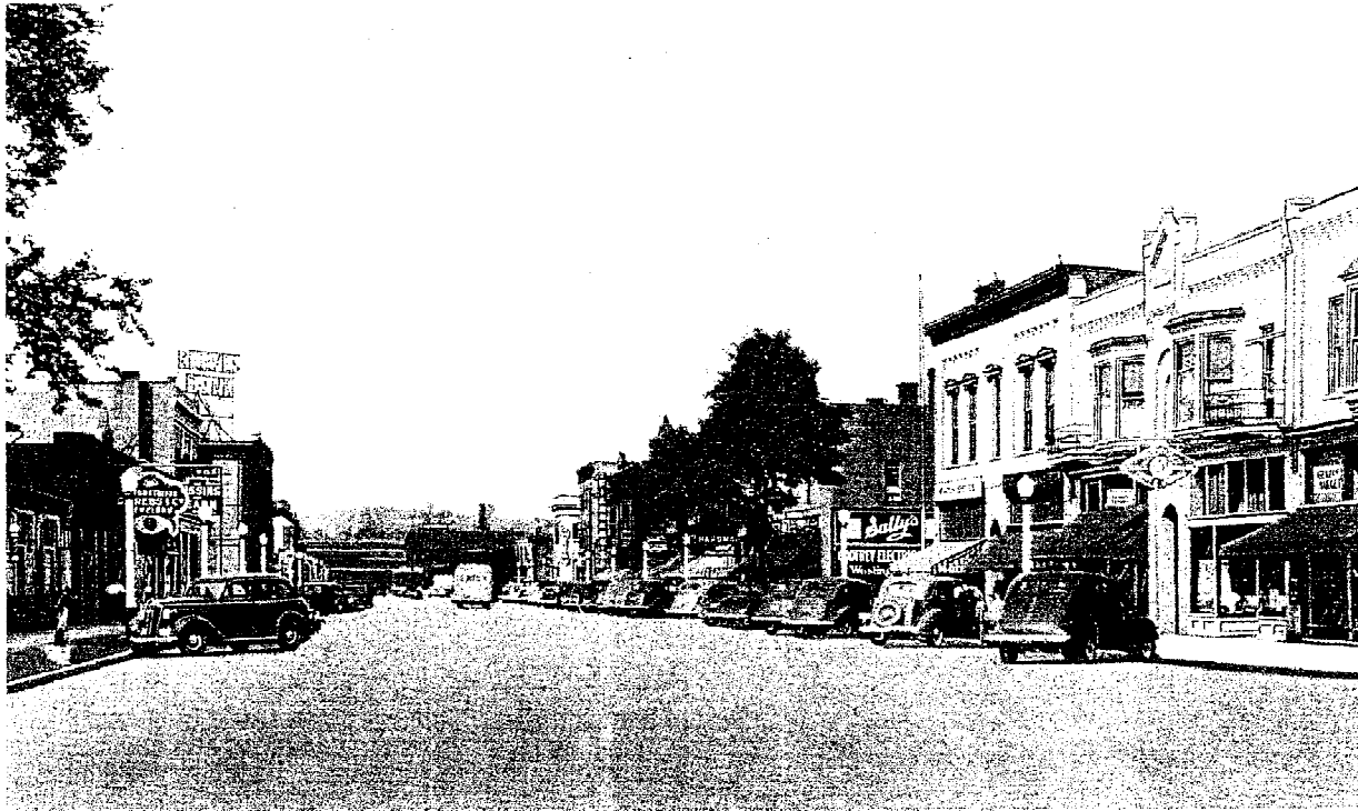
Third Street Looking West, Dover, Ohio
