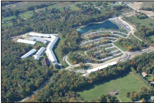
Figure 5 – Aerial View of Business Campus
