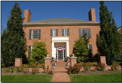
Figure 4 – Example of Residential Architecture
