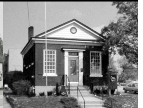
Former City Hall c. 1925
