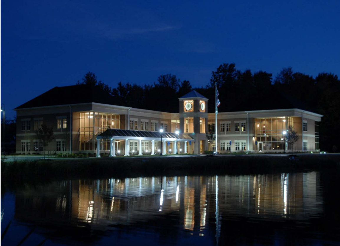
Central Administration Building
