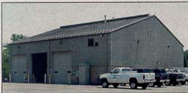
Service Garage • Built 1997
